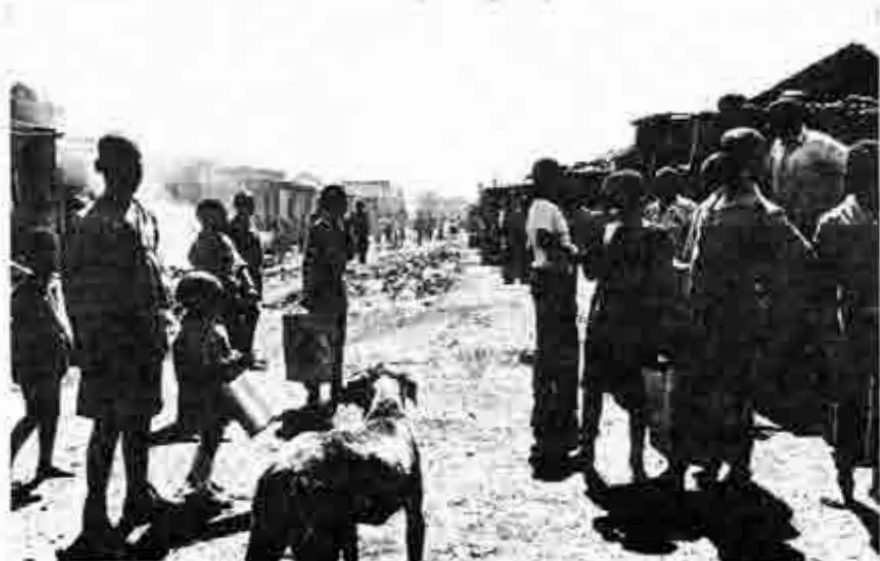
Pinville, the oldest part of Soweto. (Photo by John Seymour)
