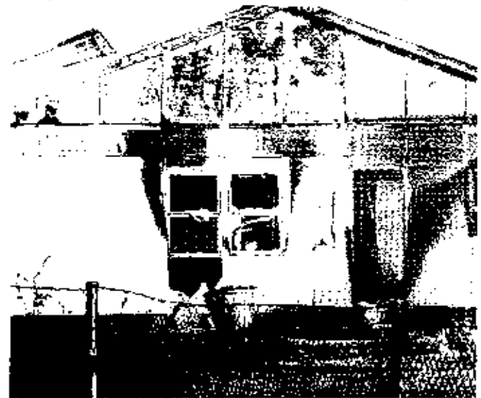
Burnt out Barclays branch in Soweto.
