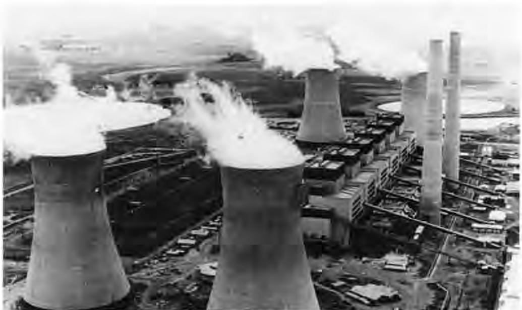
ESCOM's power station at Kriel
